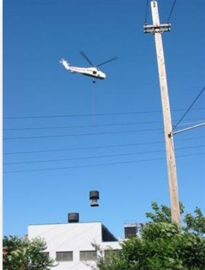
Above: Helicopter removing a vent. Below: New vent to be installed.
