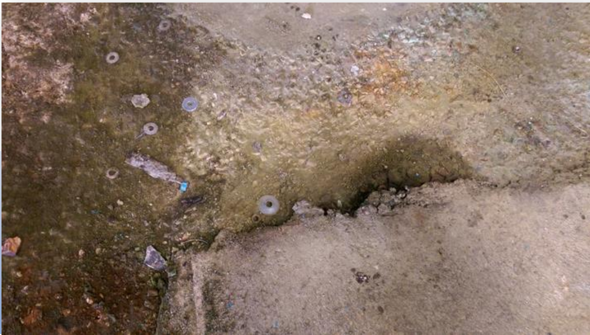
Floor conditions beneath reactors
