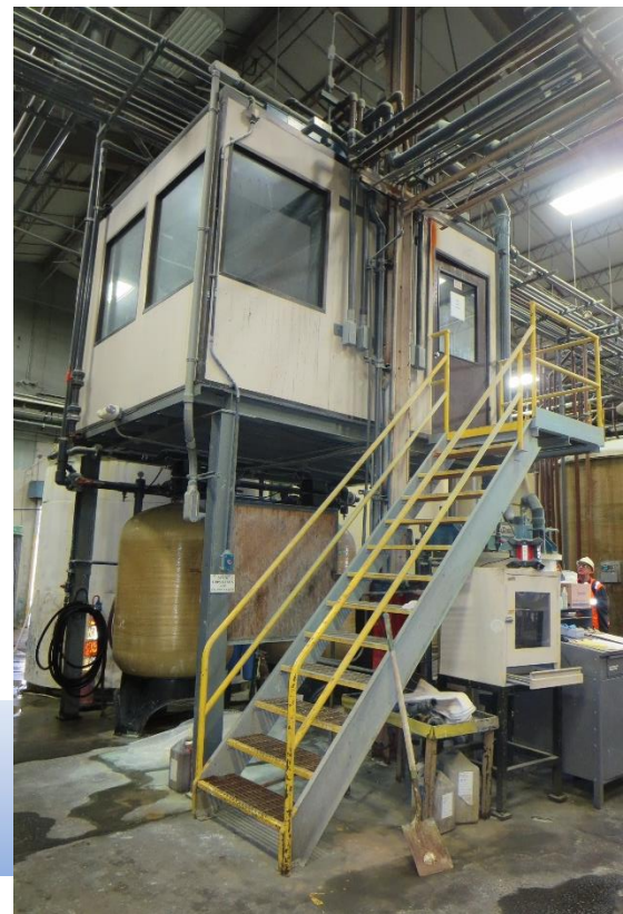
Office building requiring removal.
