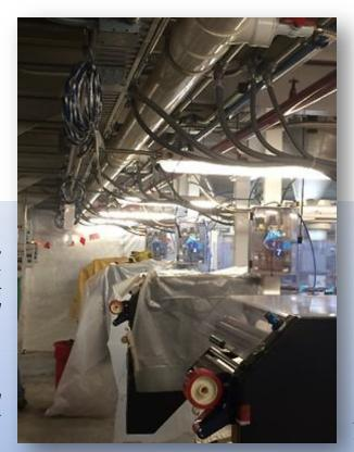
RIGHT: Temporary protective measures installed to protect equipment and process lines.
