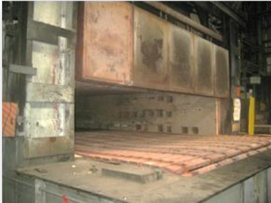
Furnace entrance before the rebuild.
