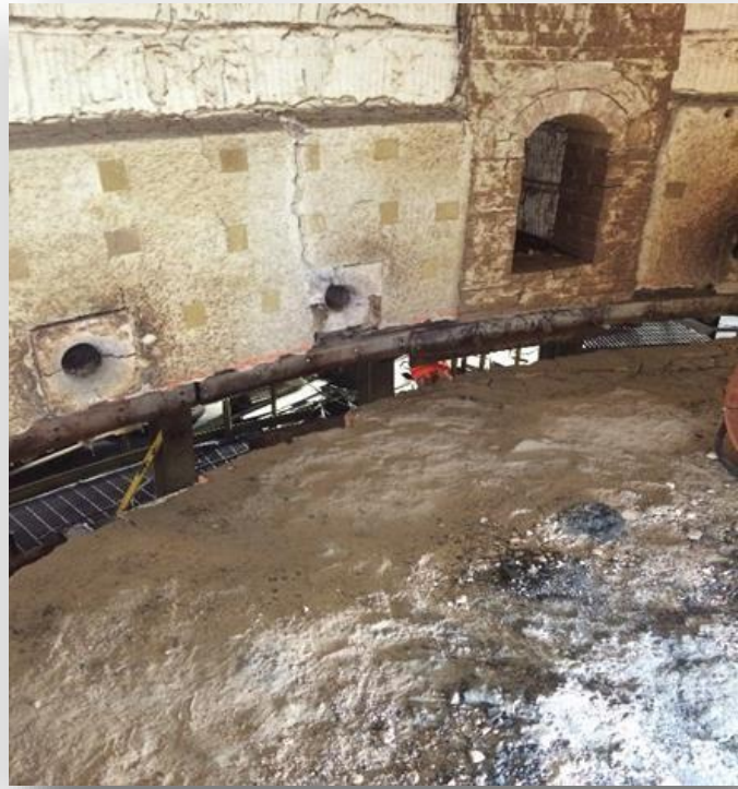
Right: Shown with wall castings, water troughs, retaining ring and water seal blades removed.
