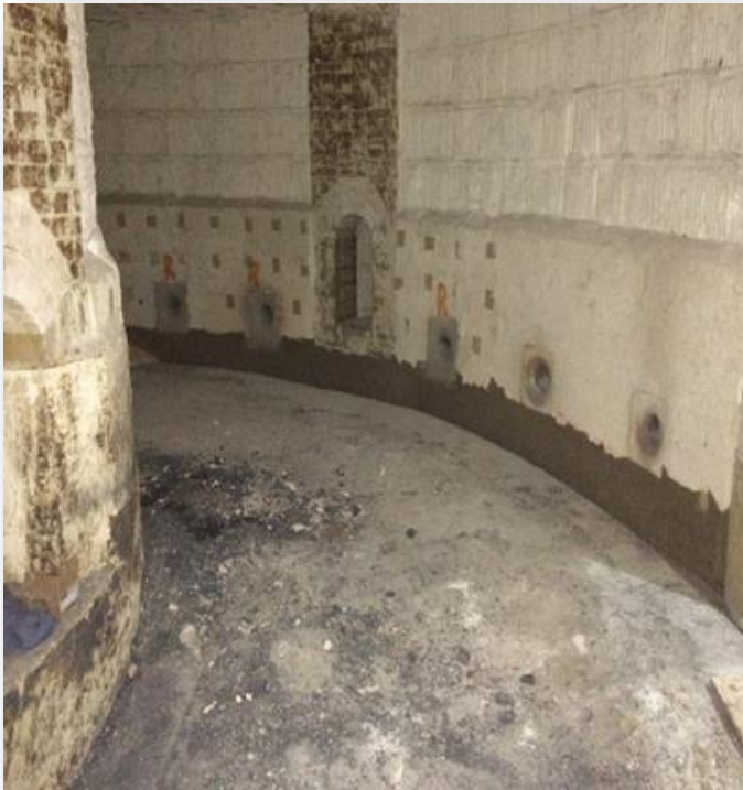
Left: Repairs to hearth and lower wall after installation of new wall castings and water troughs.
