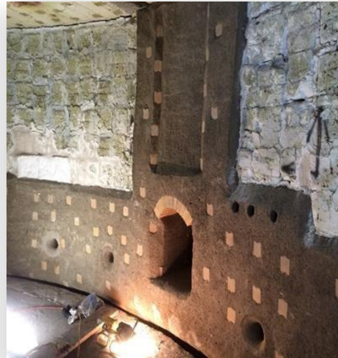
Left: Repairs to hearth and lower wall after installation of new wall castings and water troughs.
