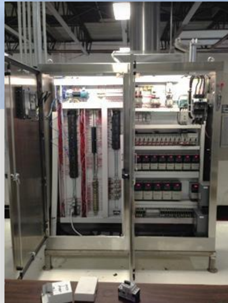
New control panel installed onsite.
