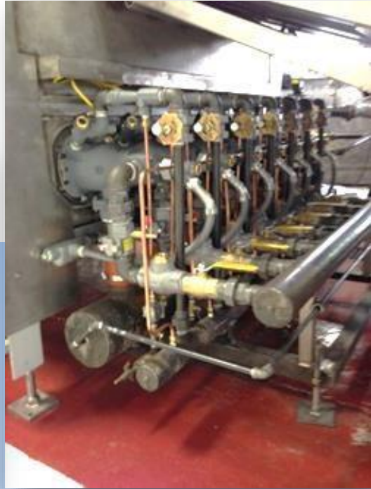
New burner system installed onsite.
