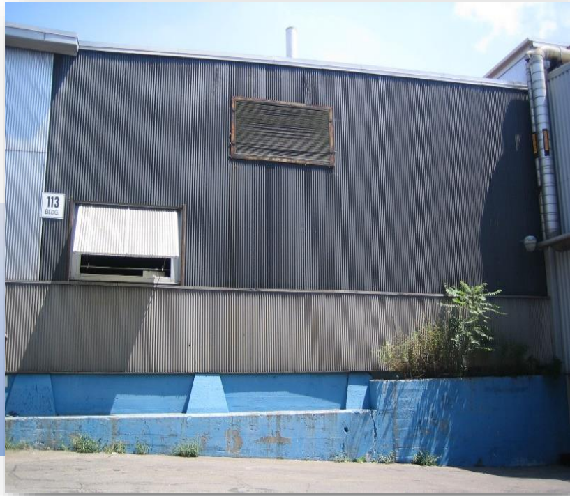
Galbestos coated siding
