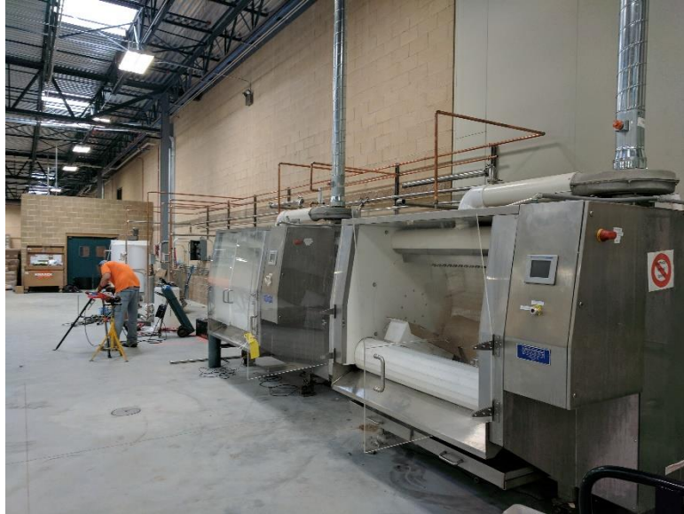
Processing area during pipe installation
